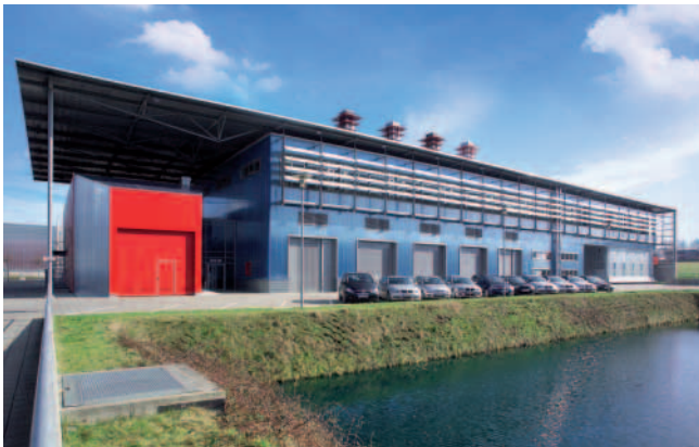
The research and development centre in Ludwigsburg with state-of-the-art test laboratories and test equipments.
